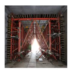
**Tunnel Formwork Traveller**
